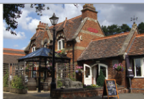
A Heritage Railway lamp stands the garden of The Brampton Hall, an extended former stationmaster's house.
